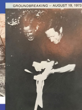
GROUND BREAKING – AUGUST 19, 1973
