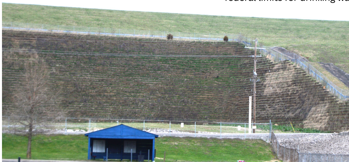
Portion of Lees Lane landfill with clay cap
