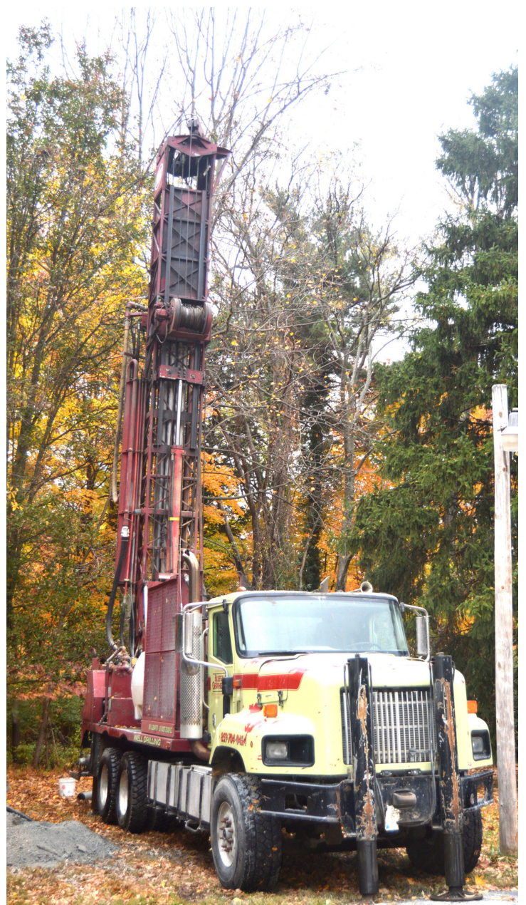
Geothermal drilling in Epiphany House’s sideyard
