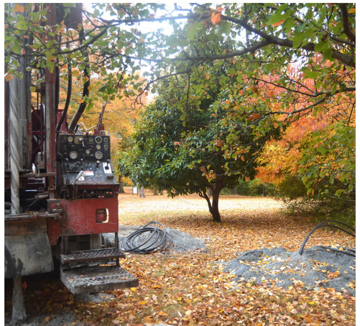
Construction site of Epiphany's geothermal well.
